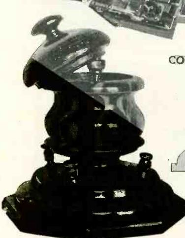
One of the prettiest as well as one of the most novel designs in radio receivers which has come to our notice recently is that shown above. Made in the form of a small urn, it is turned from two kinds of wood. The crystal detector is in the base.
