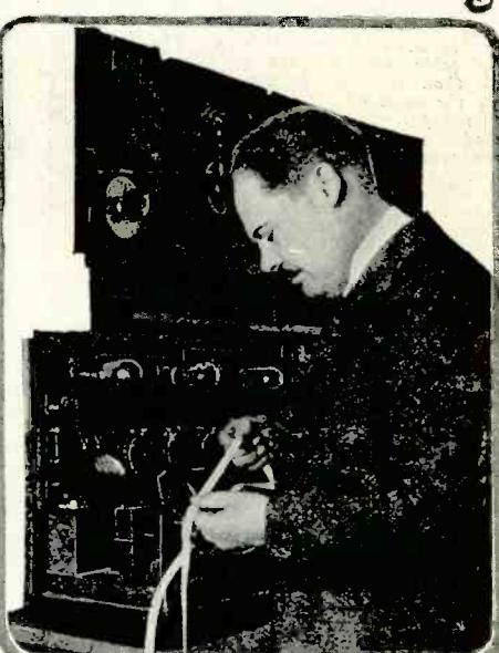
All the signals were received at the R. C. A.'s receiving station at River Head, L. I., from which the signals were passed in over land wires to the main office on Broad Street, New York City. Here they were recorded on tape moving at a given rate and calibrated in seconds. The engineer in charge is shown here reading the record breaking relay.
